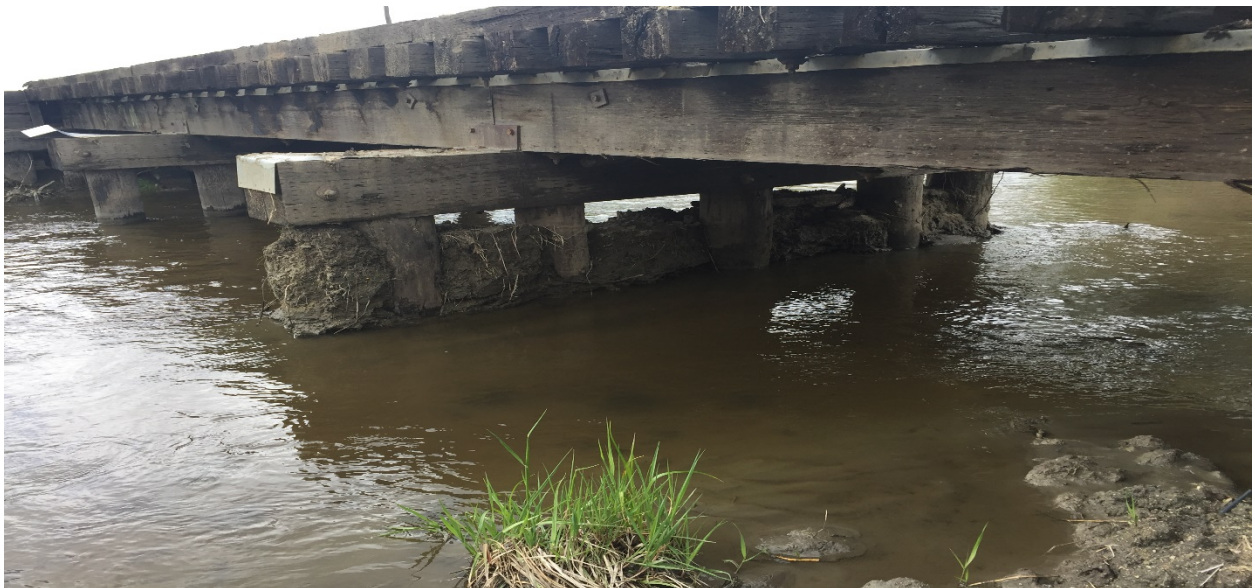
Post Sediment Removal
