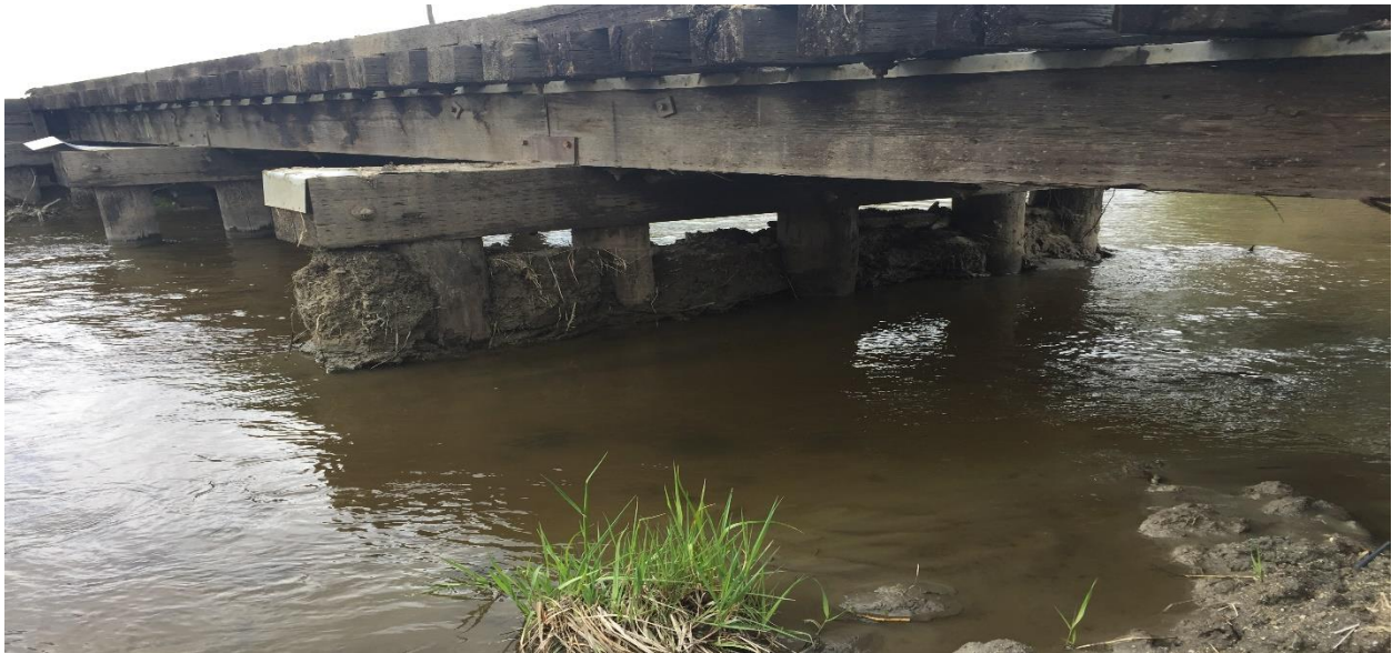
Post Sediment Removal
